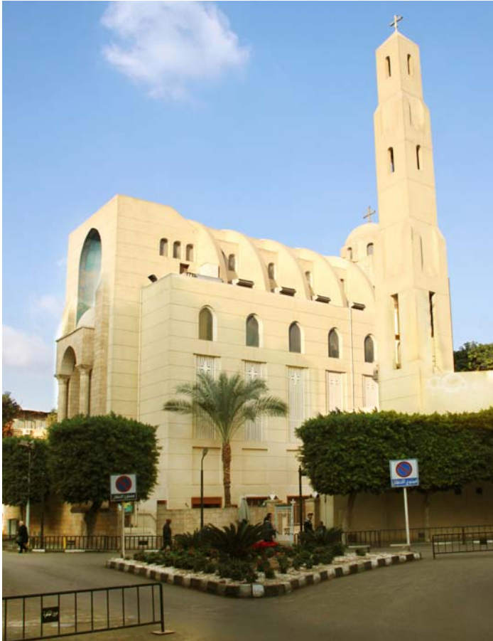
FIGURE 16.4 Church al-Mar'ashali PHOTO BY THE AUTHOR
